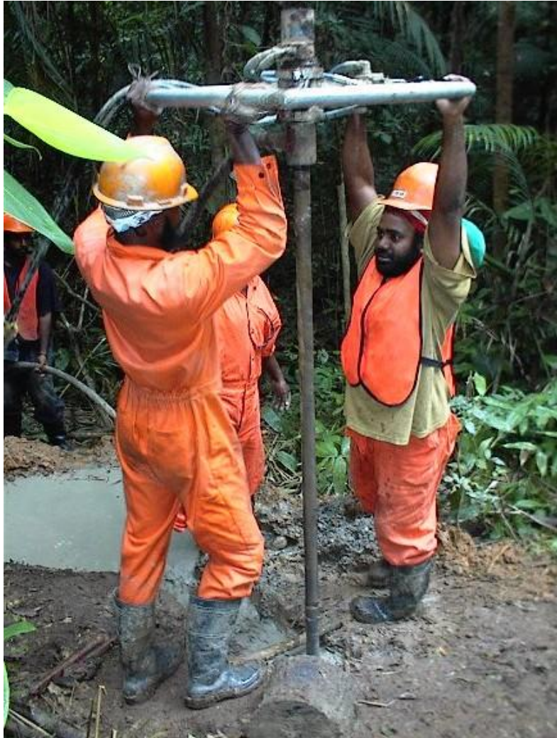
Plate 1A: Typical view of portable drilling equipment.
